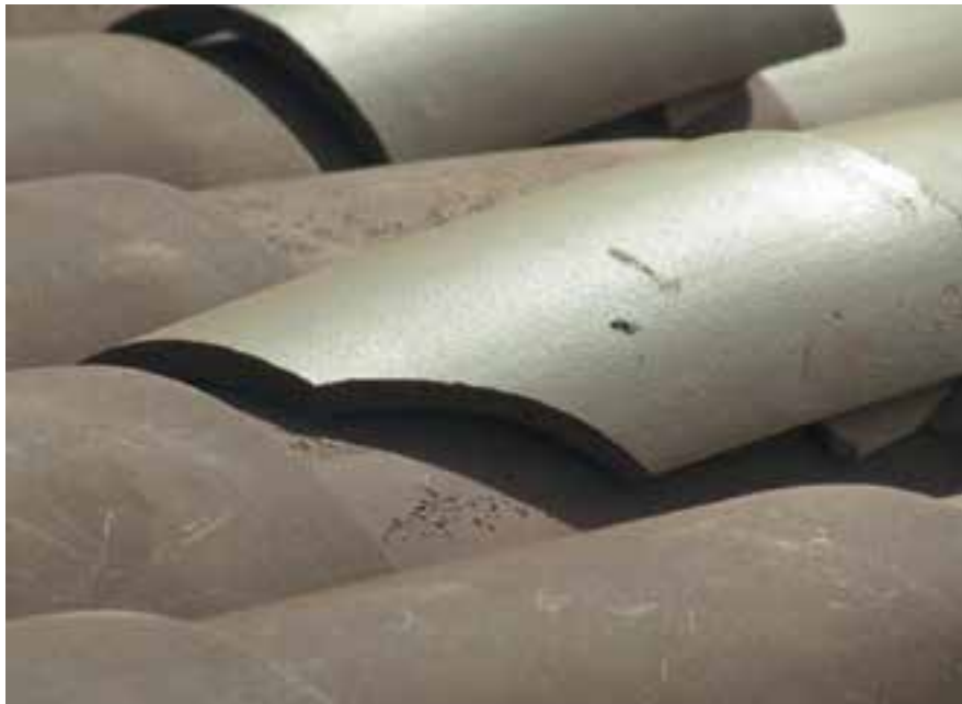
Construction inspection photo – broken roof tile.
