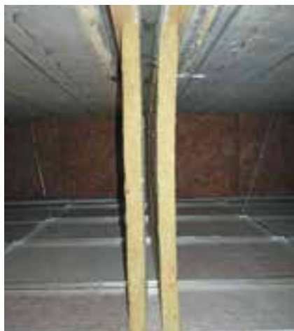
Figure 3: The intersection of a double-layer plenum barrier, ceiling system and wall. Space the plenum barrier layers apart at least 1-5/8" using a metal channel on the underside of the deck above.
