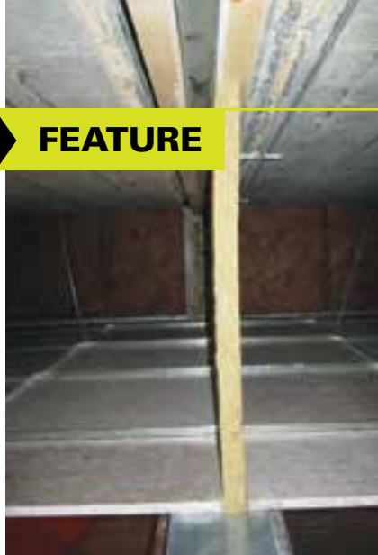
Figure 2: The intersection of a single-layer plenum barrier, ceiling system and wall. The ceiling suspension system is continuous over the demising wall. The plenum barrier abuts the top track of the demising wall. The ceiling panels are cut and lock in the bottom of the plenum barrier laterally (do not run the ceiling panel under the plenum barrier).
