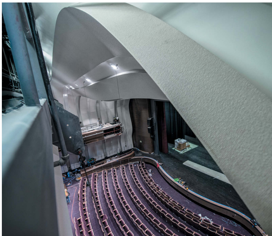
Close-up of the ribbon-framing done by Manganaro Midatlantic.
