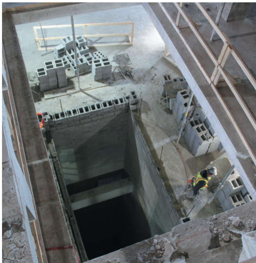
New openings created within the existing building for new stair shaft; total of eight floors tall.
