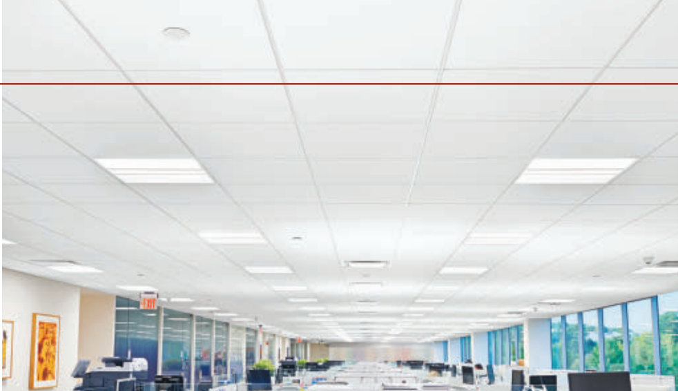
Armstrong AirAssure ceiling panels easily retrofit into existing grid systems, incorporate a gasket in their design, and have been proven to increase the effectiveness of in-ceiling air filtration by up to 40%.
